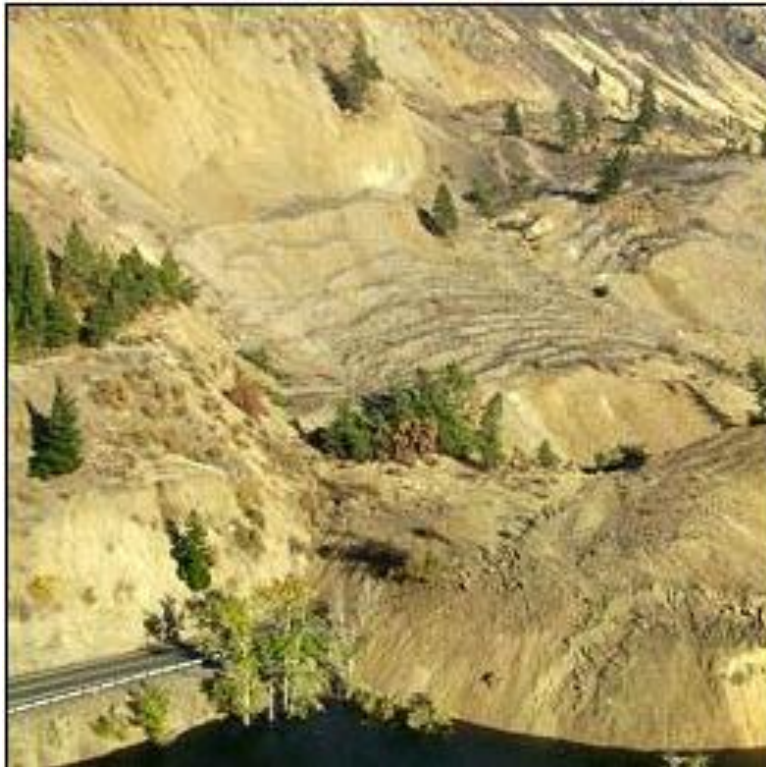
Figure 9.5 Highway 410 Near Town of Nile 2009 5 Landslide Type: Translational
